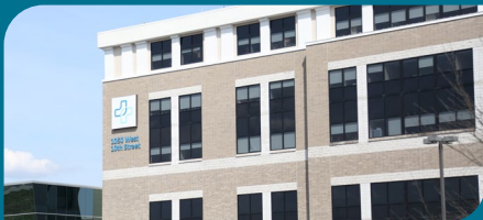
Phelps Health Medical Office Building 1050 West 10th Street Rolla, Missouri
